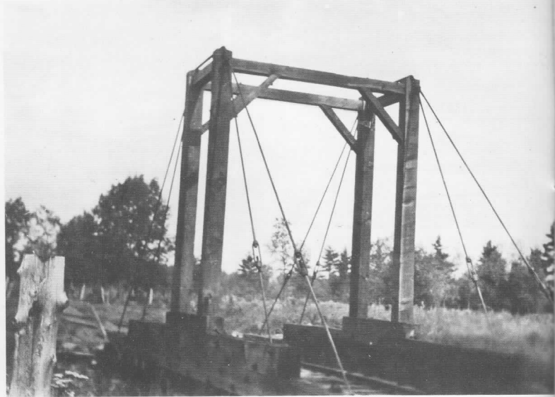
Greenwood's first turntable was a wooden affair, with a center pivot resting on rollers and circular rails. Courtesy Jack Hedlund, Soo Line Railroad Company.
